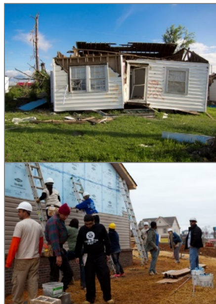
Above: A disaster-destroyed home. Below: Volunteers repair a home.
