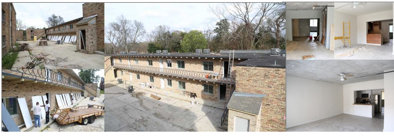
Rental units in Louisiana being repaired under Multi-Family Lease and Repair to house eligible applicants.
